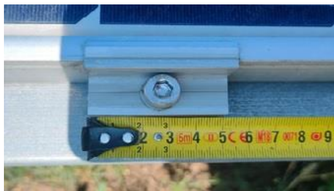
Fig.4 Measuring the distance of the mounting clamp from the edge of the module
