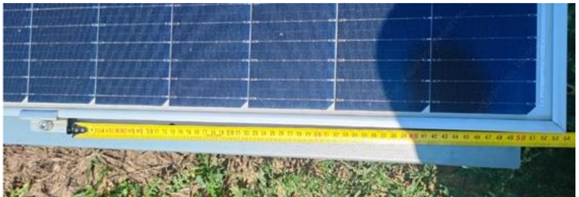
Fig.4 Measuring the distance of the mounting clamp from the edge of the module
