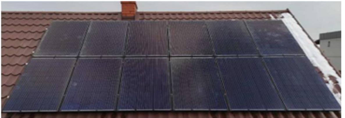
Fig. 3 Photos taken on a cloudy day. Visual differences caused by dirt and moisture.
