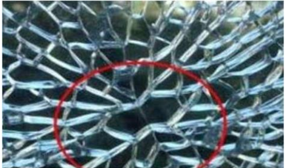
Fig.1 Spontaneous cracking - a "butterfly-shaped" point
